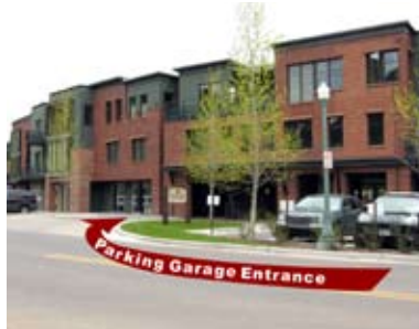
North Facade with Parking Garage Entrance
